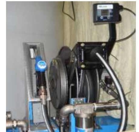
25' Hose Reel, Filter, Pulse Out Meter
