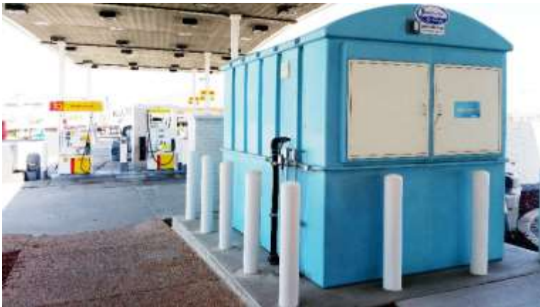
Insulated & Heated Supplying Multiple Remote DEF Dispensers
